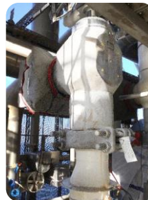
INSTALLATION AT TROLL C
