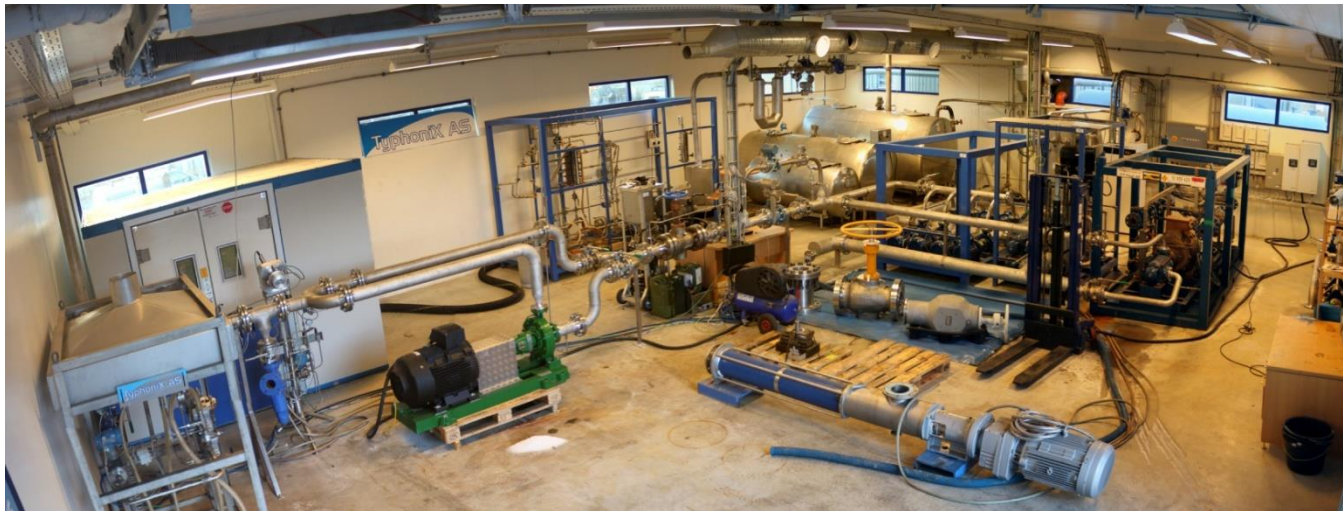
3-Phase Lab testing facilities
